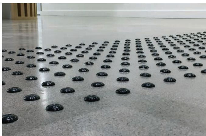
Black PVD coated domes installed on tile flooring.
