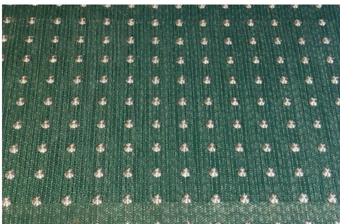
Stainless steel concentric ring domes installed on carpeted flooring.
