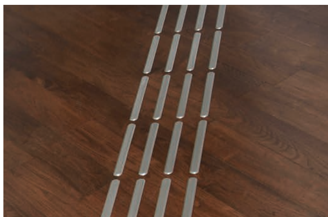
Linear grooves wayfinding bars installed on hardwood flooring.
