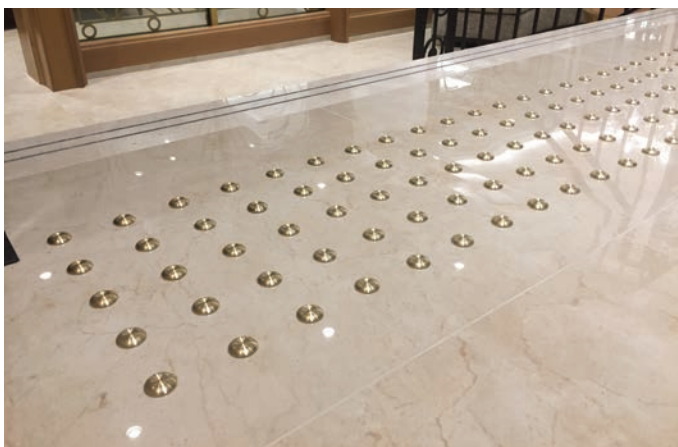
Brass truncated domes installed on marble flooring.
